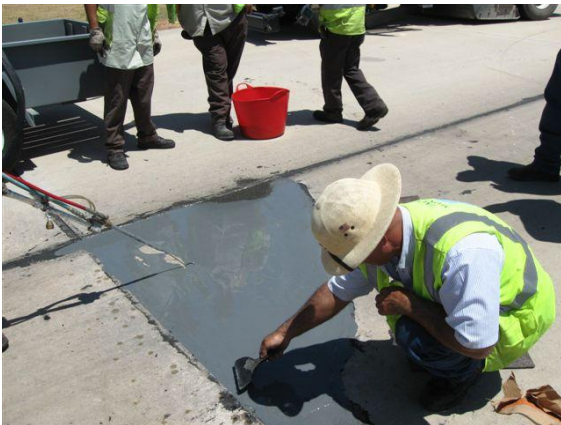
Corner spall returned to service in 1 hour at San Antonio Airport
